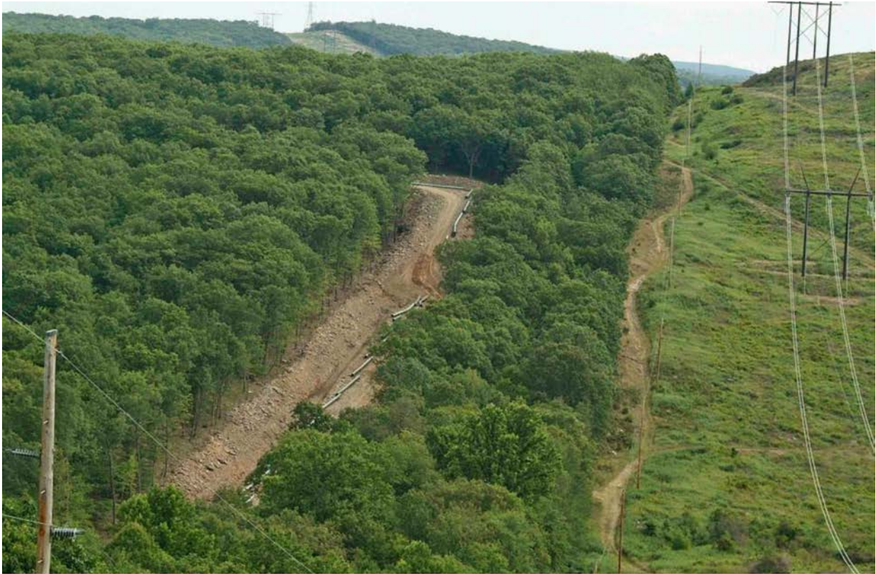
Image from PennEast powerpoint showing a right-of-way through woods.
