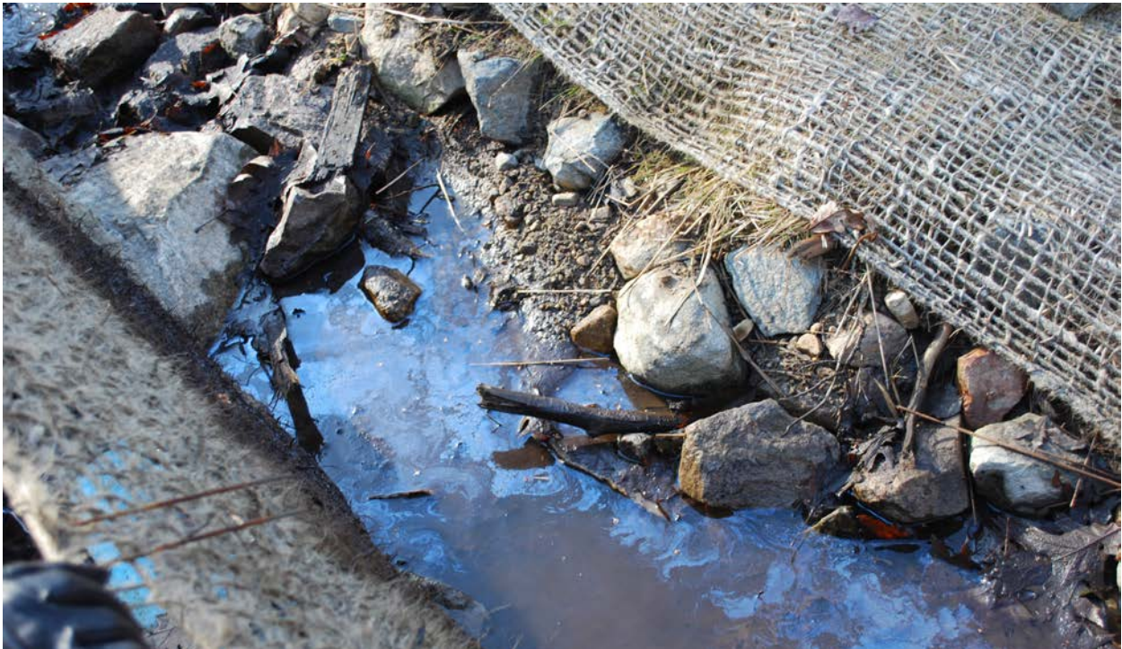
Image taken by North Jersey Pipeline Walkers of pipeline construction sites.
